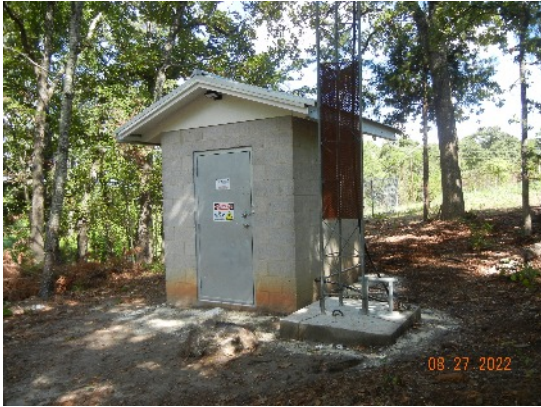
UAARC 2M Repeater on Simpson Mt.
