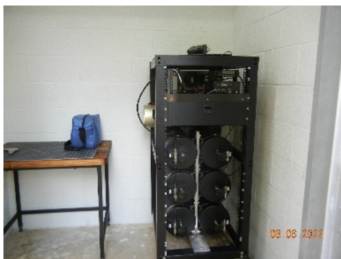
Repeater mounted in building.
